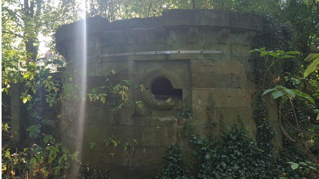
Plate 18A-2: A Grade II*listed mid-18th century bastion, pierced through to be utilised as a defensive structure during World War II.
